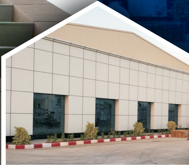
ACP for Wall Cladding
